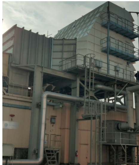
New Airfilco filter house
