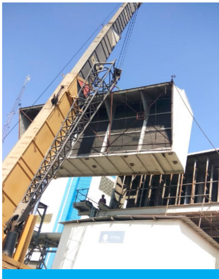
Dismantling original filter house
